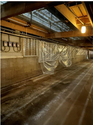
Fans sealed with plastic and house wrap
